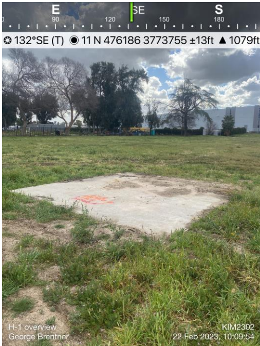
Photo 2: Overview of Concrete Foundation (Not a Historical Resource; View SE)
